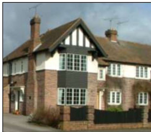
The stained effect UPVC windows do not reflect the materials and style of the originals and harm the symmetry of the semi-detached pair. Carefully designed UPVC windows in the same colour and subdivisions of the original windows can have a less harmful effect on the character of the conservation area.
