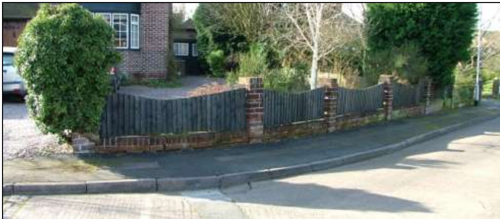
Original brick wall with piers and concave elliptical curve to top of riven oak infill
