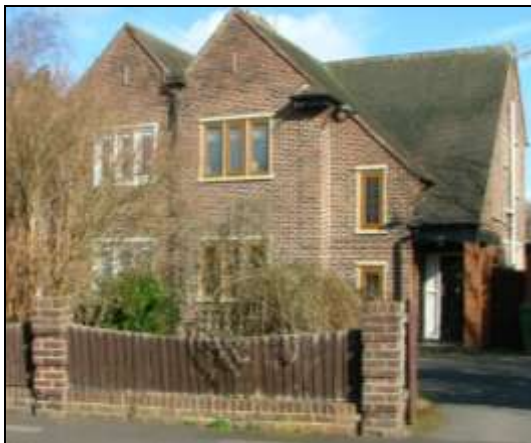
The stained effect UPVC windows do not reflect the materials and style of the originals and harm the symmetry of the semi-detached pair. Carefully designed UPVC windows in the same colour and subdivisions of the original windows can have a less harmful effect on the character of the conservation area.
