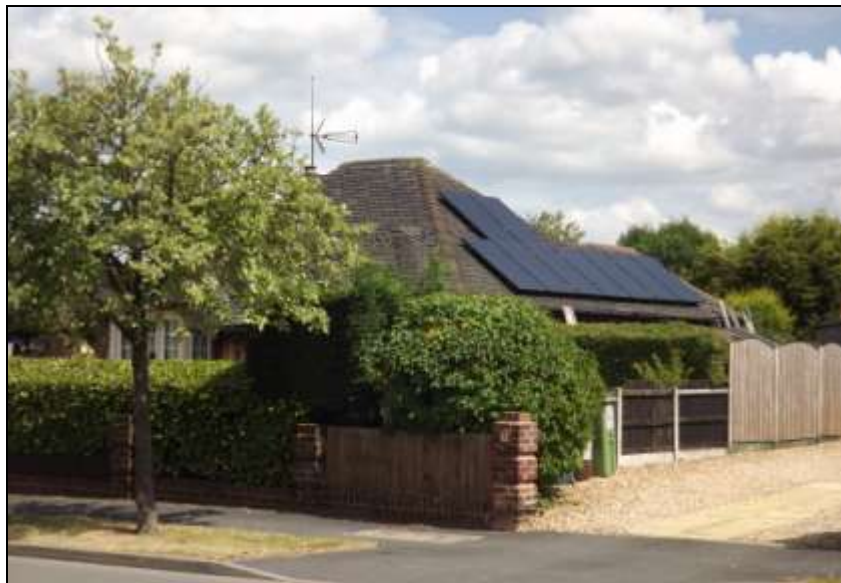
Solar panels can dominate the appearance of roofs
